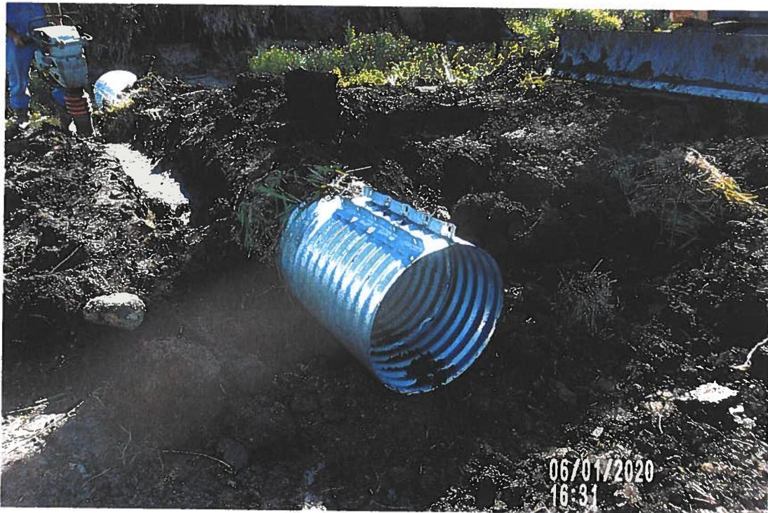
PICTURE # 3624 IS LOOKING SW SHOWING CREW JUMPING JACK COMPACTING LOOSE SOIL ON SIDES OF PIPE WITH 24" CMP BAND IN PLACE.
