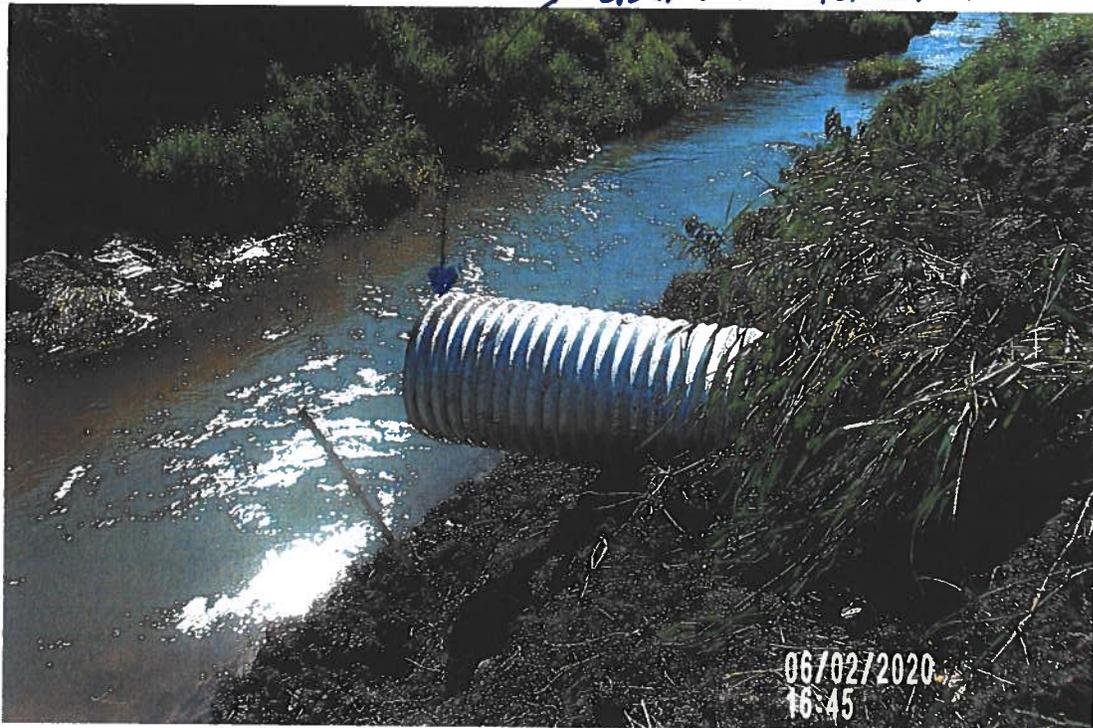
PICTURE # 3645 IS LOOKING AT NEW 24" CMP OUTLET AT DRAINAGE
