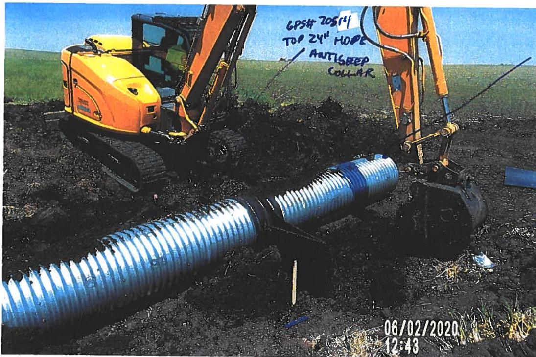
PICTURE #3634 IS LOOKING NE AT 2 BANDS AND 5 BOLTS FASTENING LOWER ANTISEEP AND PARTIAL UPPER ANTISEEP.
