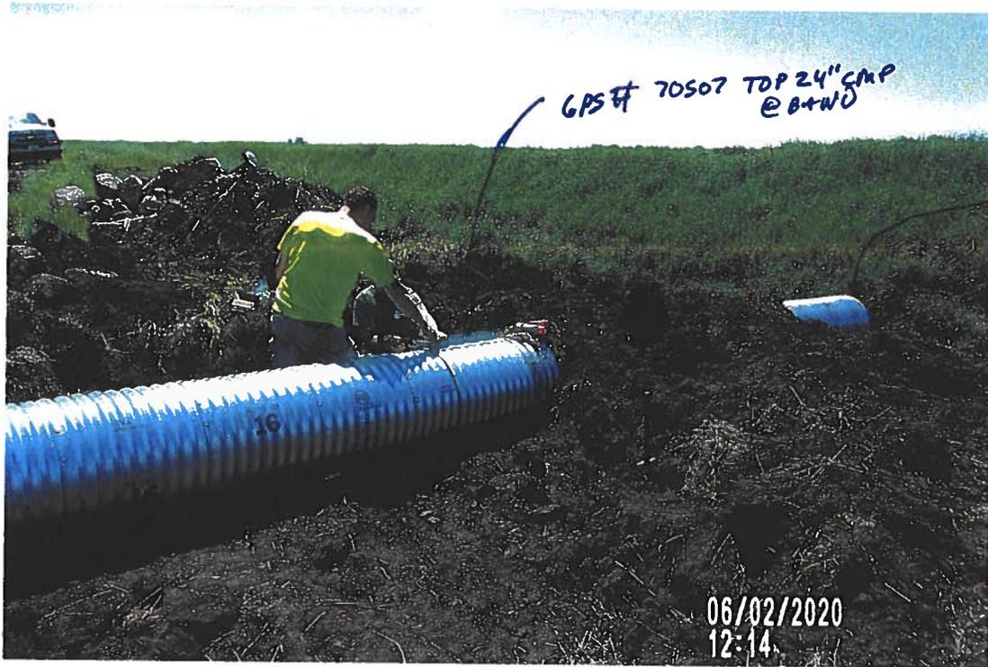
PICTURE# 3633 IS LOOKING NW SHOWING 24" HDPE ANTISEEP COLLAR IN PLACE WITH 2 BANDS AND 5 BOLTS FASTENING LOWER ANTISEEP AND PARTIAL UPPER ANTISEEP HDPE COLLAR ONE EAST SIDE
