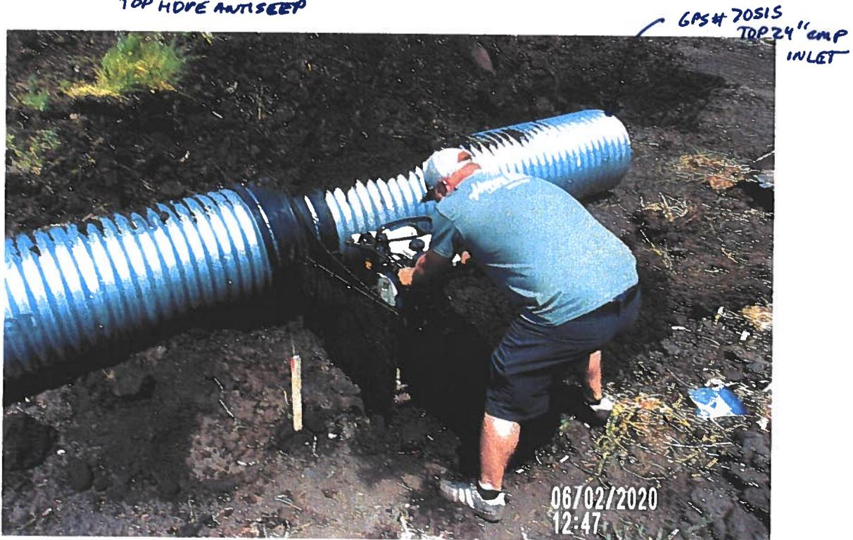
PICTURE # 3635 IS LOOKING NW SHOWING CREW JUMPING JACK COMPACTING SOIL AROUND 24" HDPE ANTISEEP COLLAR.
